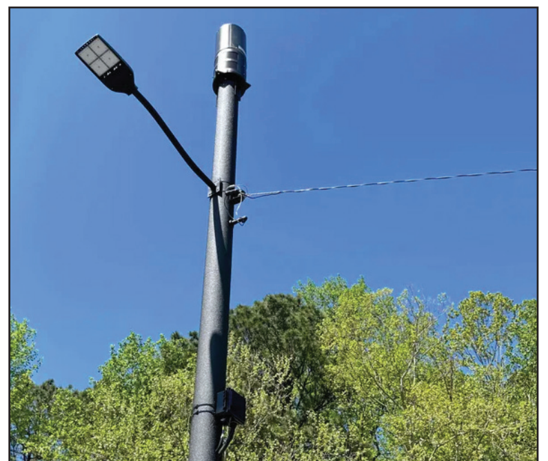
Fifty-foot-tall, small-scale cell towers could be key to providing reliable, readily accessible cell phone service to critically underserved rural areas in Vermont. Judiciously placed, the relay towers can significantly improve the “shadowing” effects of Vermont's mountains and copious forestation that cause cell phone signals to drop or be altogether inaccessible in many instances.
